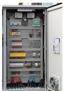
Image 2: Electrical enclosure temperatures in Greece can rise to 60°C or more – the HIMatrix modules with expanded temperature range used here are designed for temperatures up to 70°C.
