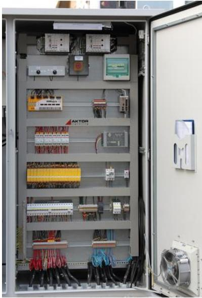
Image 2: Electrical enclosure temperatures in Greece can rise to 60°C or more – the HIMatrix modules with expanded temperature range used here are designed for temperatures up to 70°C.
